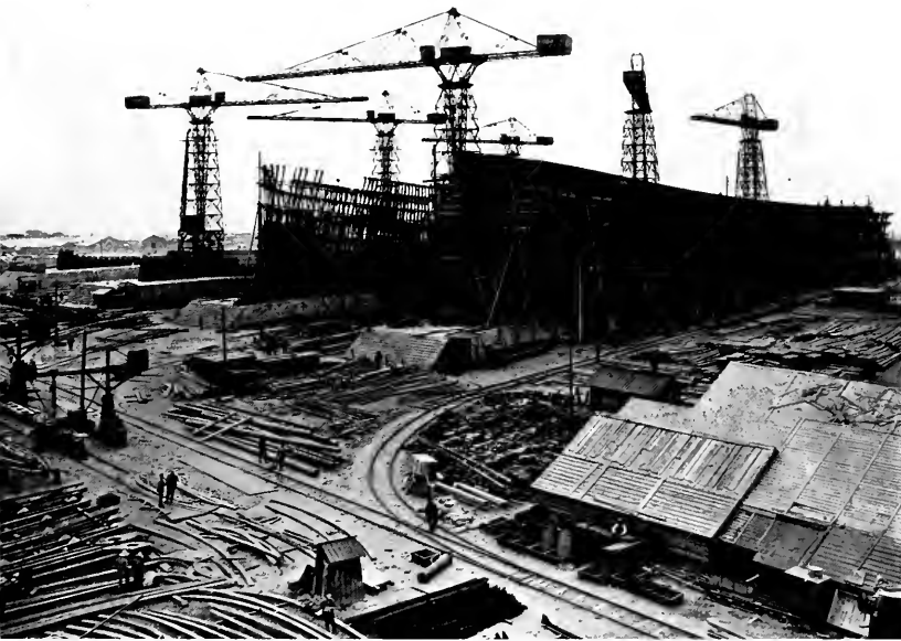
View looking towards the upper ends of building berths.
